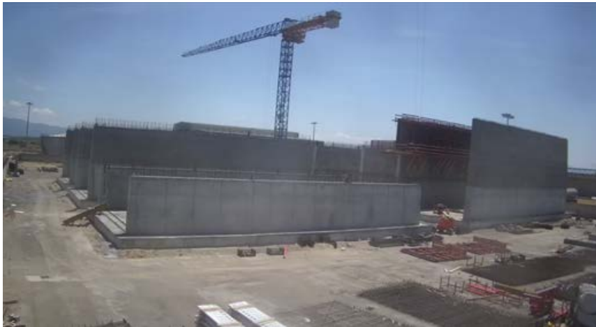
Higas LNG receiving terminal in Sardinia
