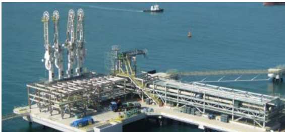
Aqaba Terminal Infrastructure
